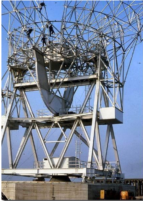
Assemblers at work in 1982 to complete the support structure of the primary mirror of the 32m diameter parabolic antenna at the Medicina radio astronomy station. Credits: INAF-IRA
