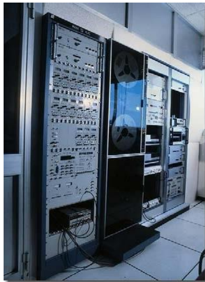
The VLBI MKIII terminal of the Medicina station. On the left, the devices for converting the observation frequency to medium frequency, the 14 Base Band Converters, and the apparatus that prepares the signal before being sent to the magnetic tape recorder on the right. Credits: INAF-IRA
