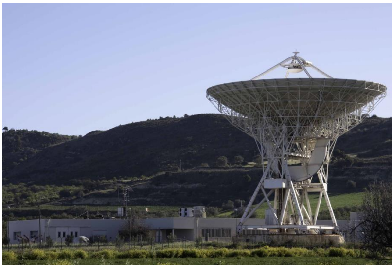
The 32 m diameter antenna inaugurated on October 28th, 1988 near Noto (SR). To the left of the antenna the buildings of the radio astronomy station. Credits: INAF-IRA
